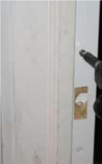
3. While ensuring the Fix-A-Jamb component remains properly positioned shim secure it into place with the attached screws. No pre-drilling is required with the screws for the Interior FIX-A-JAMB piece. For the Exterior FIX-A-JAMB piece, it may be necessary to pre-drill a hole, using a 11/64" drill bit.
