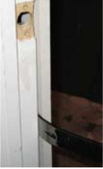
1. Carefully remove door trim molding around the area of the jamb needing repair. This is best done with a pry bar or the back end of a claw-foot hammer. This material can and should be reinstalled upon installation completion.
